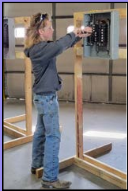
Garrett Spevacek installs a breaker box. Photo contributed by Randy Robertson.
